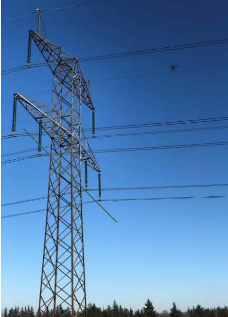
A drone in the sky inspecting power lines. Photo: Geopartner Inspections.
